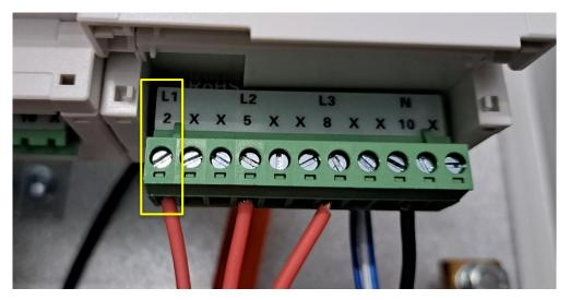
The power supply must come from the consumer side of the main switch, and before all loads and inverters.
