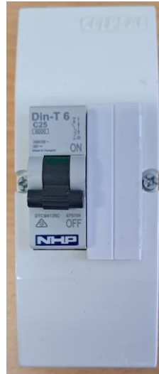
Picture 4 – MCB in a 2-pole enclosure
