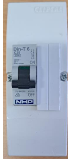
Picture 4 – MCB in a 2-pole enclosure
