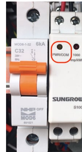
Figure 9: PWR/COM light on the S100 Sungrow meter
