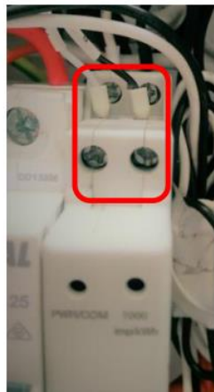
Pictures 1 & 2 – S100 connections to Hybrid inverter. White = A and Black = B
